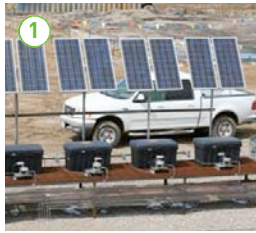
1 USA Pipeline-Service Sunpumper
